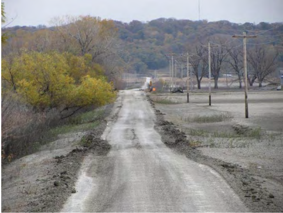
Figure 144. Gravel surface on TS2 at the time of testing (Picture taken on 10/26/11)
