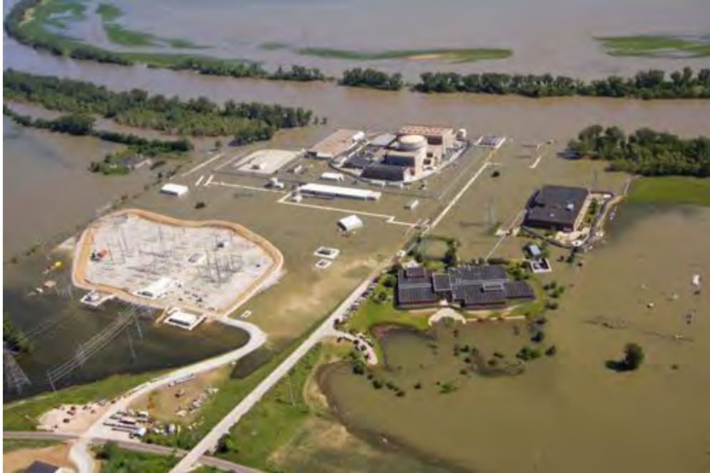
Figure 12. Aerial photo of the flooding near the Fort Calhoun nuclear power plant near Blair, Nebraska on June 17, 2011 (Image Courtesy of Omaha Public Power District)
