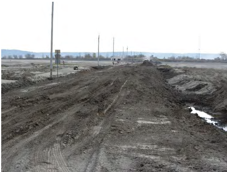
Figure 53. Reconstruction of a gravel road washed away during floods and deposited with silt and sand– Fremont County (Photo taken on 10/26/11)
