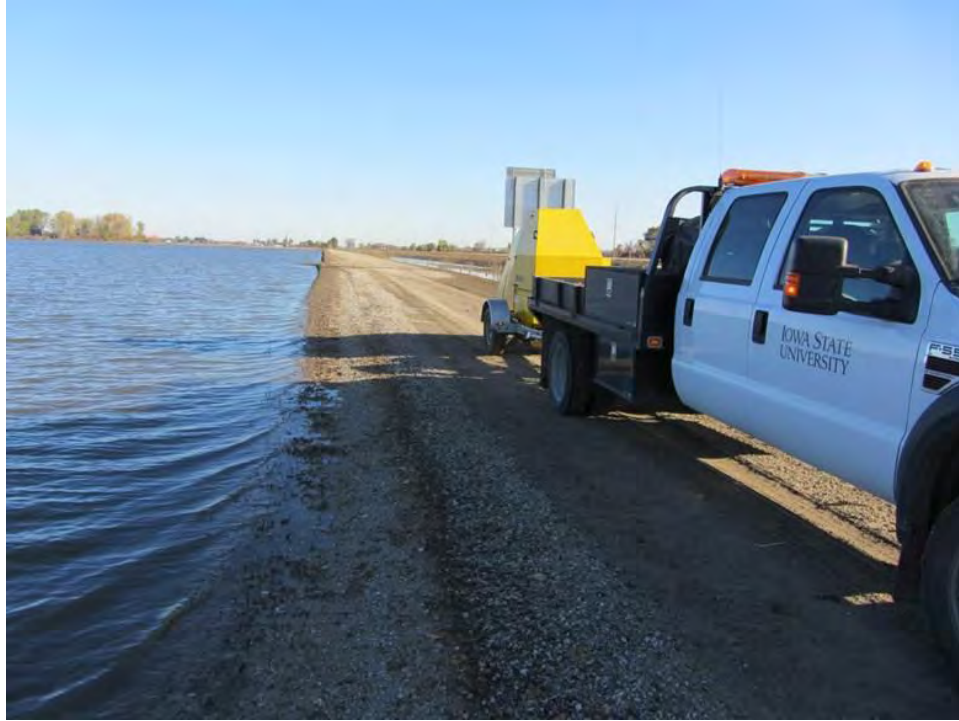
Figure 90. FWD testing on TS5 with floodwater up to the edge of the road (Photo taken 9/23/11) – Pottawattamie County
