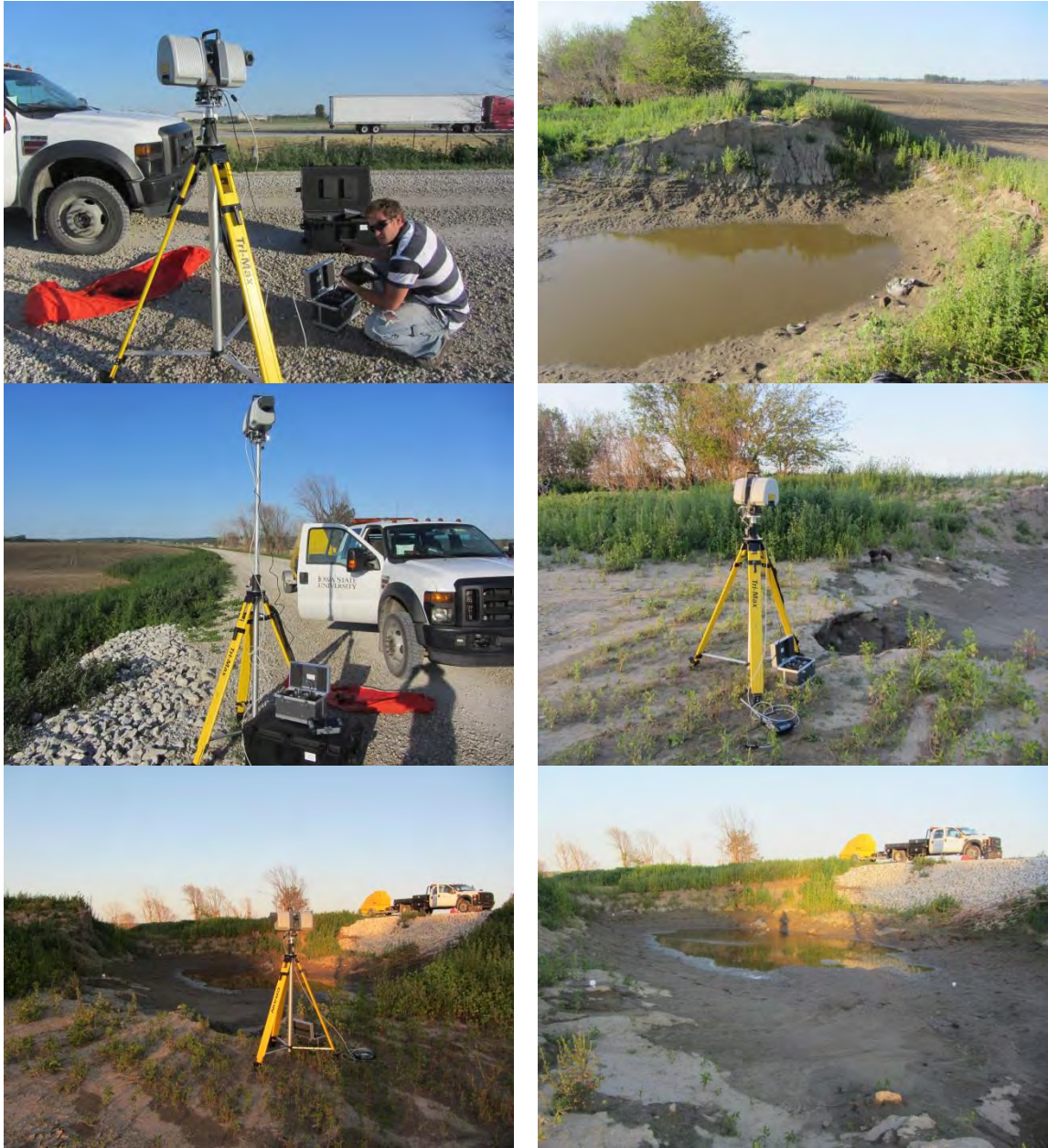
Figure 98. 3D laser scan setup at the levee breach site on TS5 145th St. – Pottawattamie County
