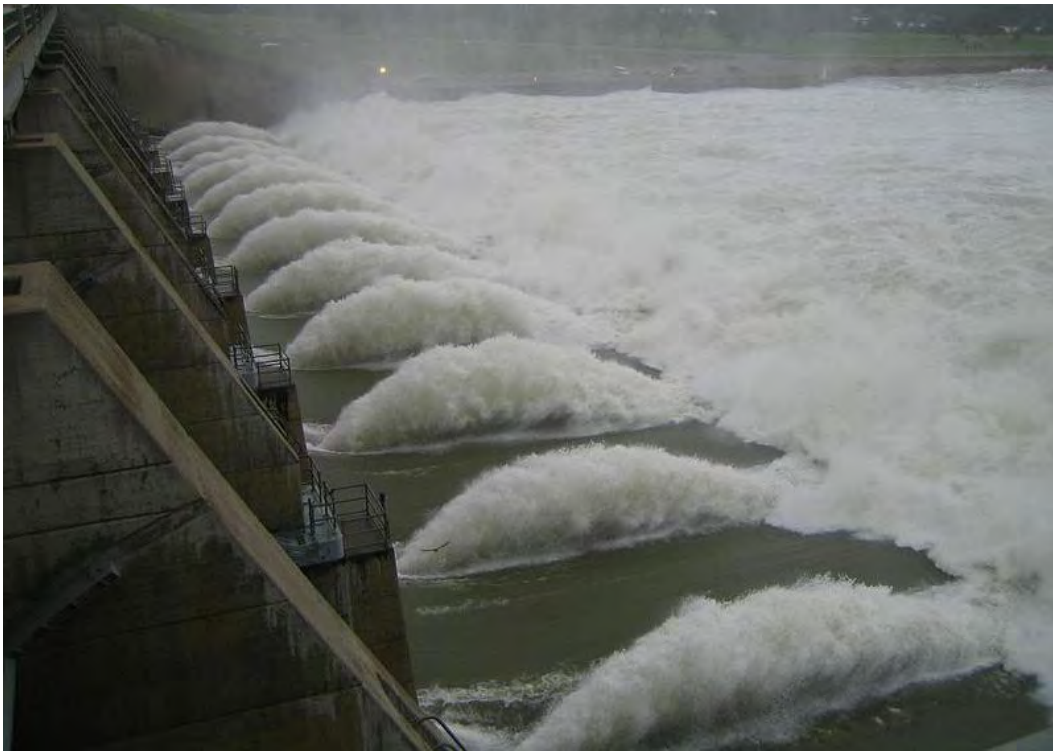
Figure 9. Gavin's Point dam releases 150,000 ft 3 /s of runoff volume on June 14, 2011 (Image Courtesy of Jay Woods, USACE)
