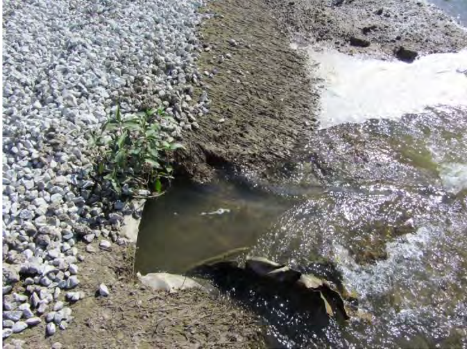
Figure 112. Replacement gravel cover over culvert (Picture taken on 9/23/2011) – Pottawattamie County
