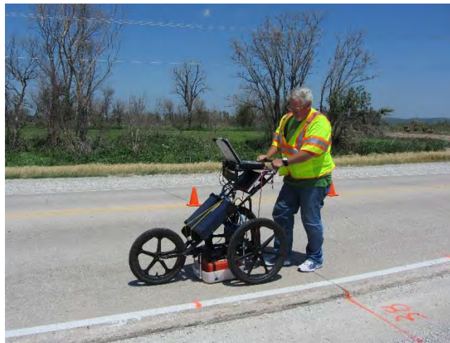
Figure 25. Ground penetrating radar scanning using GSSI SIR-20 data acquisition system
