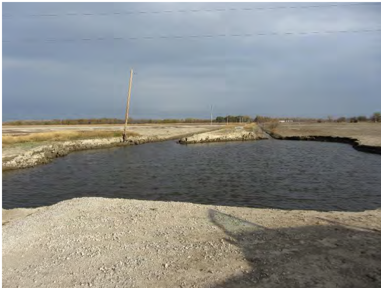
Figure 51. Full breach of a gravel road (about 100 m (330 ft) long) – Fremont County (Photo taken on 10/26/11)
