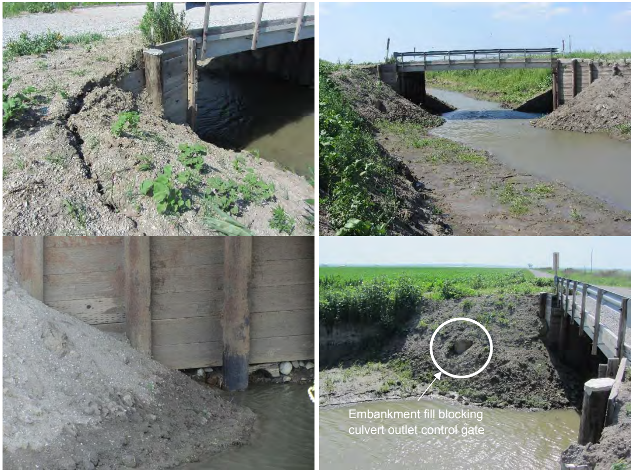
Figure 135. Bridge conditions on TS1 on 6/9/12 – Fremont County
