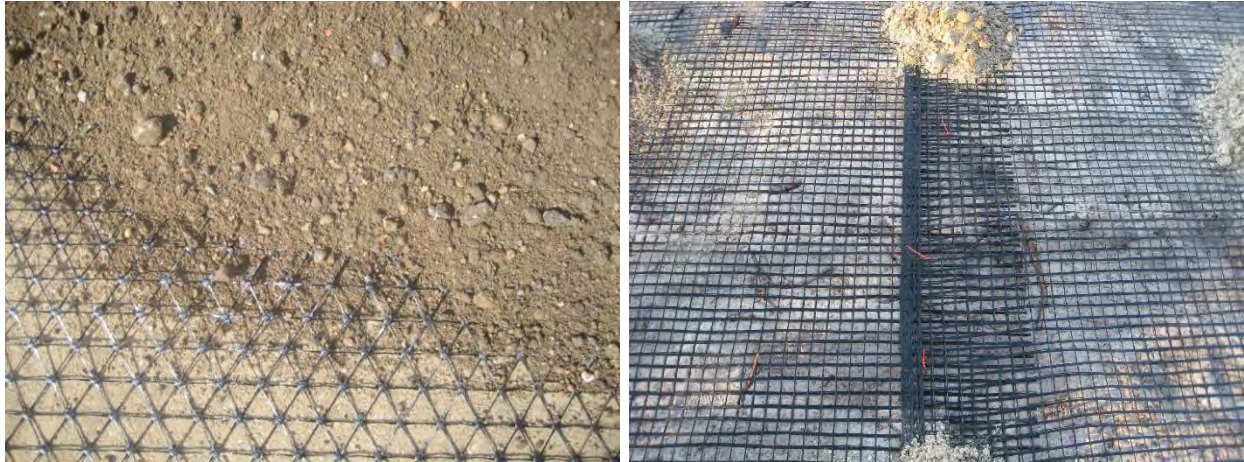
Figure D34. Triaxial (left) and biaxial (right) polymer geogrids placed on the subgrade
