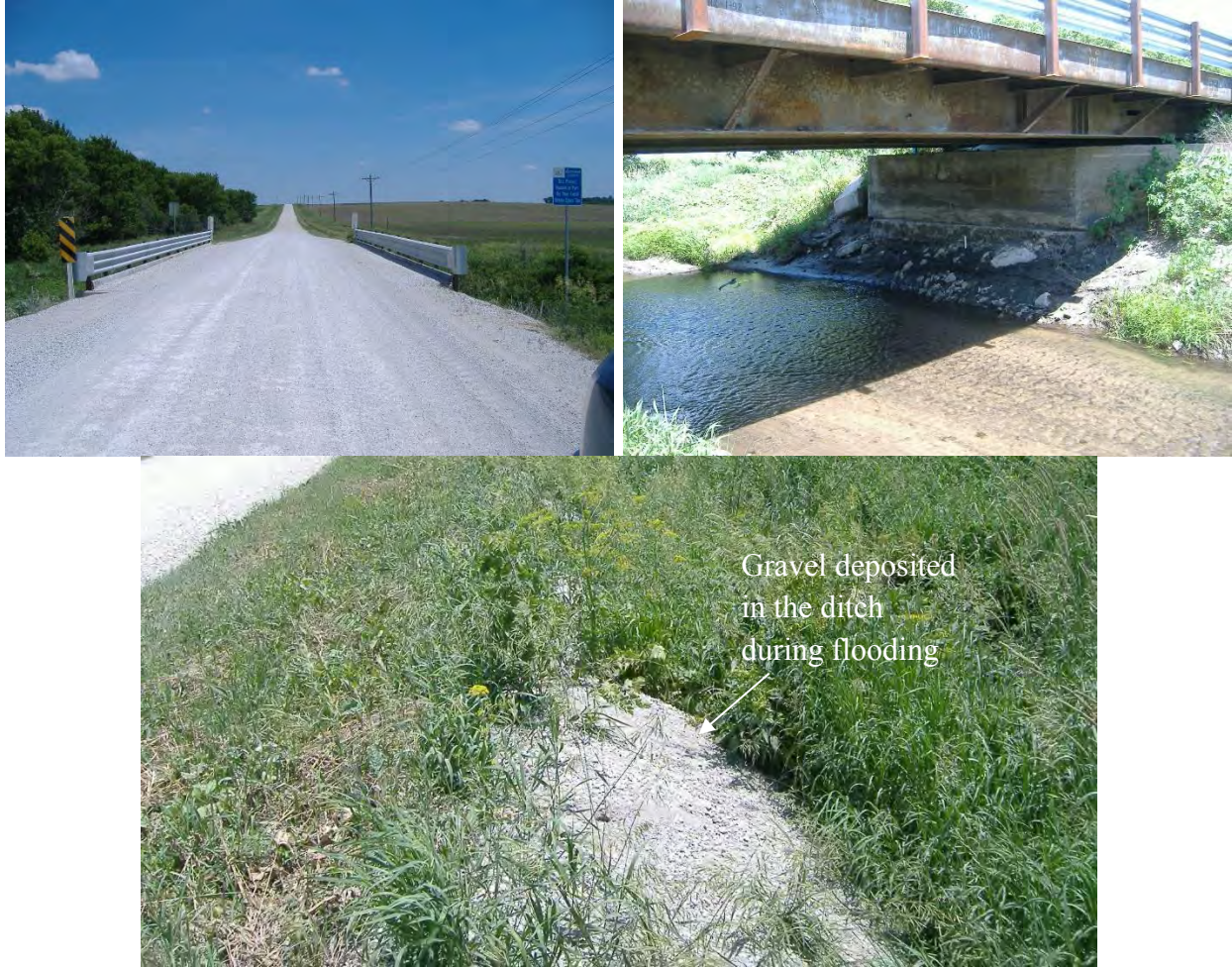
Figure D42. Pictures of a bridge site in Buchanan County (250 th Street) after flash flooding occurred in May 2013
