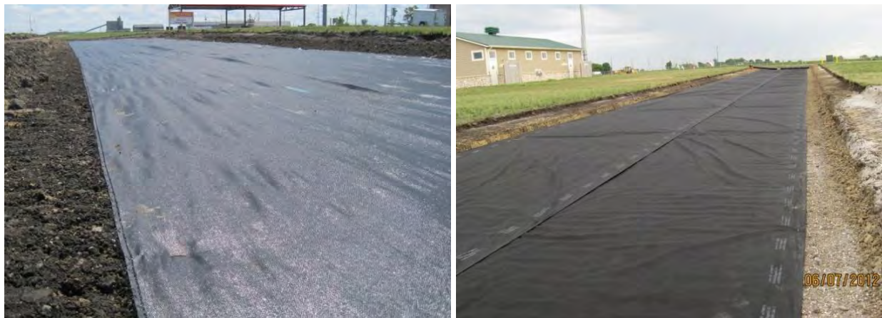
Figure D33. Woven geotextile (left) and non-woven geotextile (right) placed at subgrade/aggregate layer interface
