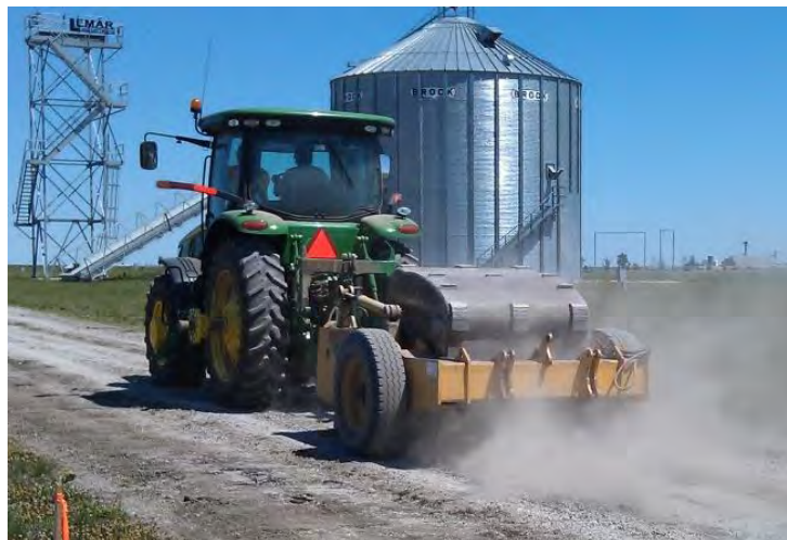
Figure D35. High energy impact roller (equipment by Impact Roller Technology, Plattsmouth, Nebraska)
