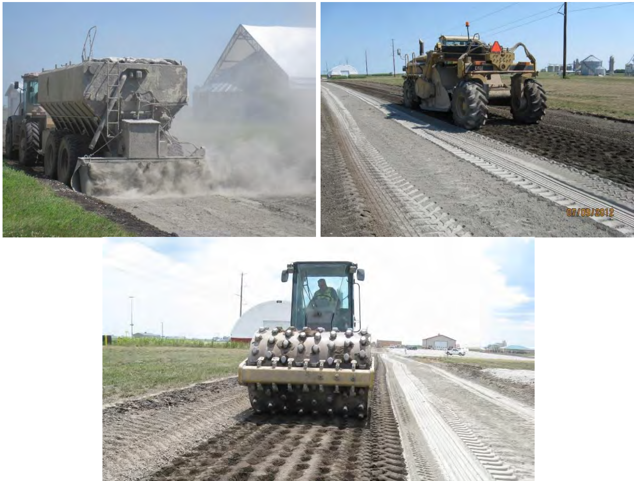
Figure D30. Photos showing typical chemical stabilization process
