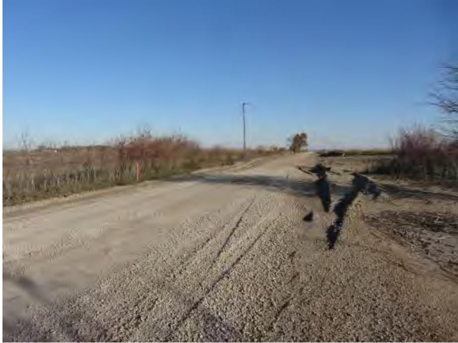
Figure 155. Newly placed gravel near a culvert at about 4700 m station on TS2 (Picture taken 10/27/11)
