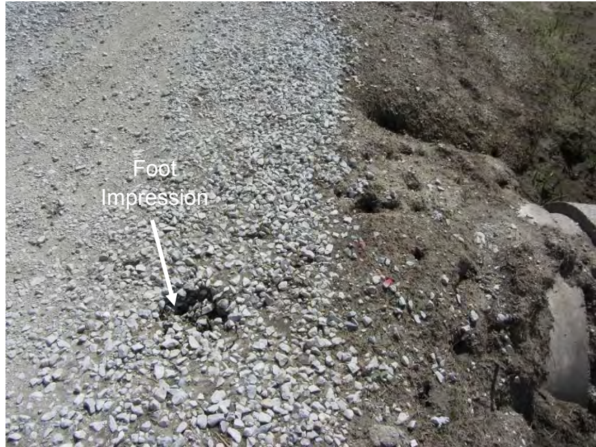
Figure 92. Loose backfill material around culvert replaced after flood waters receded on TS5 (Photo taken on 4/5/12) – Pottawattamie County
