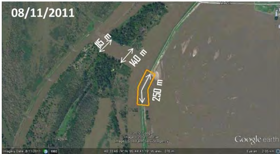
Figure 36. Levee breach in southern part of Fremont County (images updated on 6/9/10, 7/17/11, and 8/11/11)
