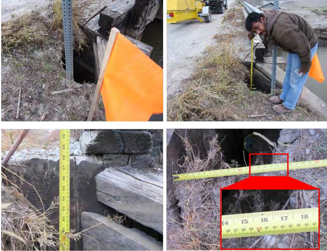
Figure 146. Void behind the west abutment wall due to erosion of backfill material at TS2 bridge (Pictures taken on 10/26/11) – Fremont County
