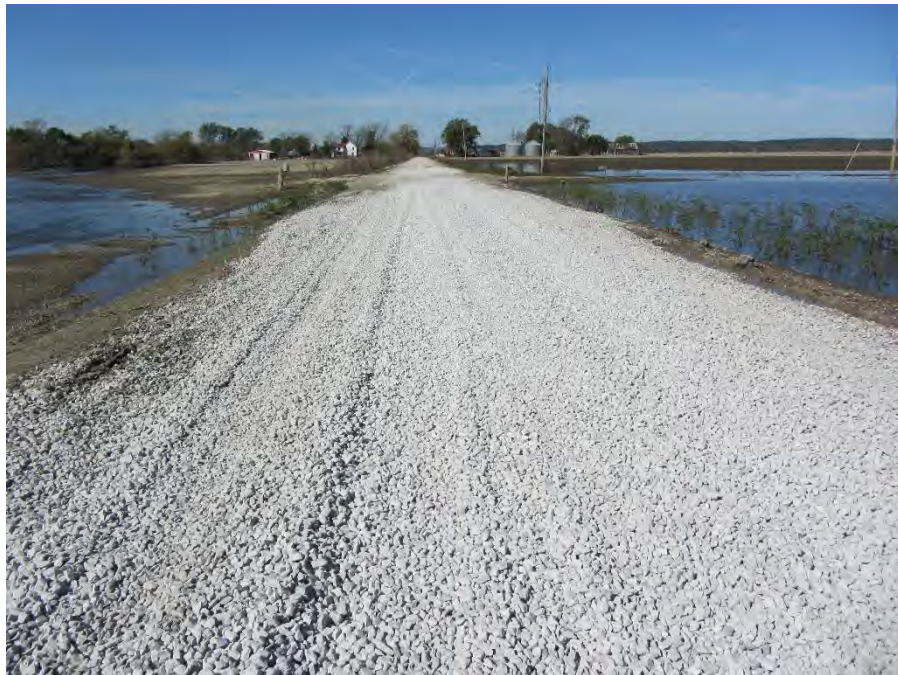
Figure 113. Location of newly placed gravel on TS6 over a metal pipe culvert (Picture taken on 9/23/11) – Pottawattamie County
