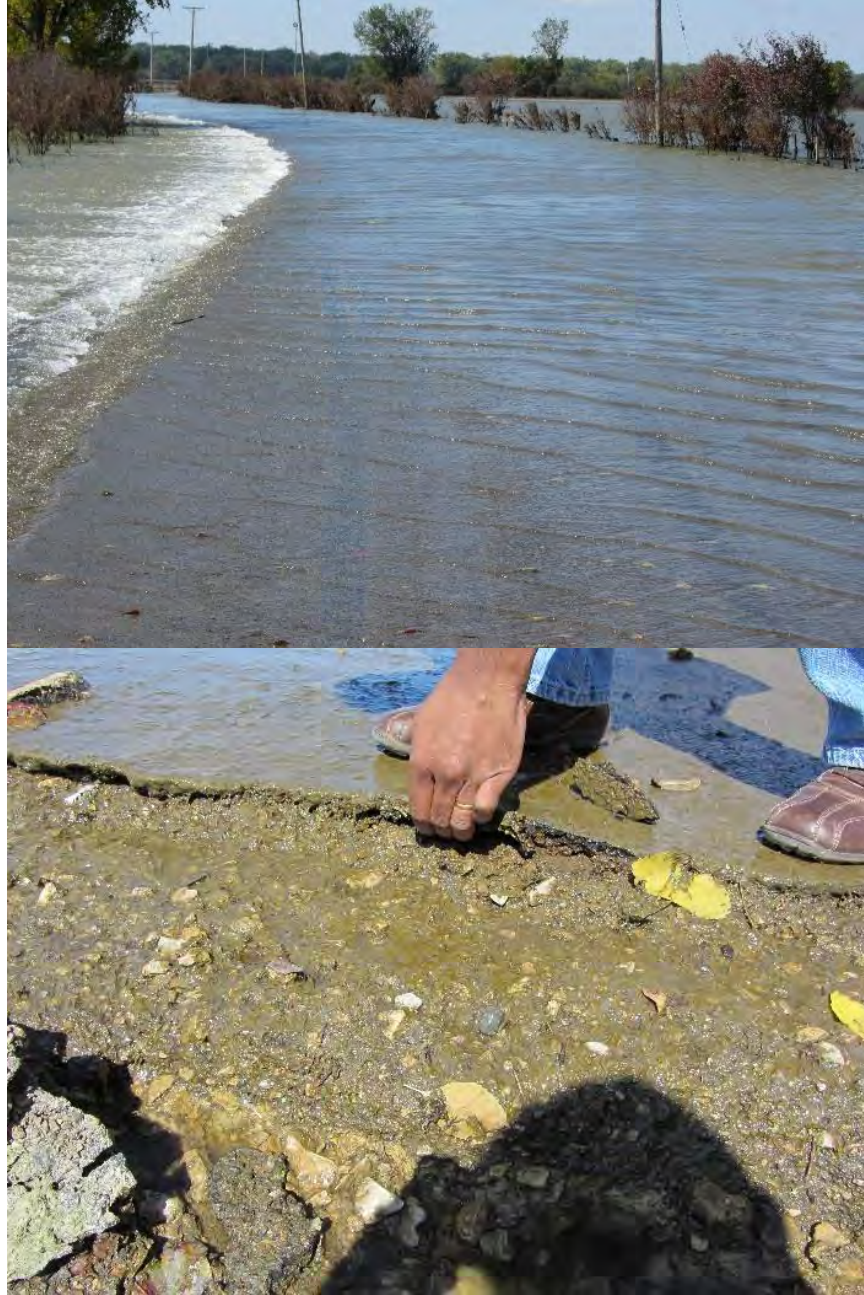
Figure 120. Water overtopping Desoto Avenue on 9/21/11 and delamination of chipseal coat at the surface (Pictures taken on 9/21/11) – Pottawattamie County
