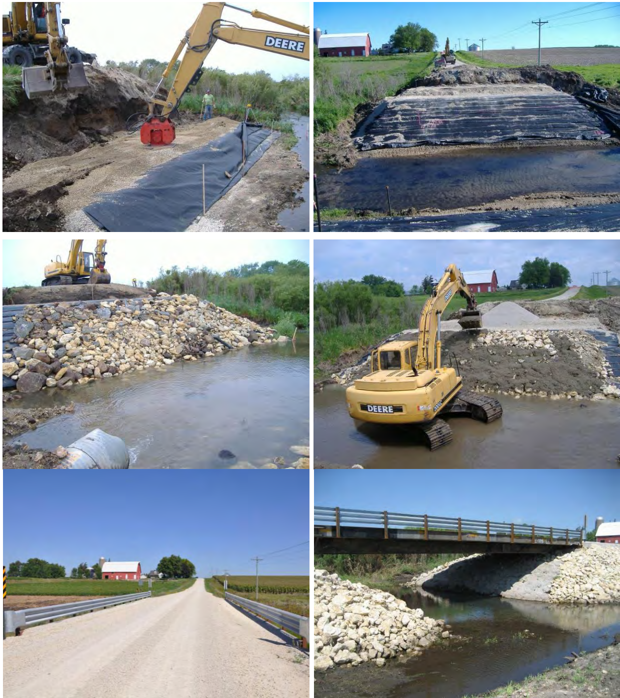
Figure D39. Pictures of a bridge site in Buchanan County (Olympic Ave.) during construction of GRS fill in bridge abutments, placement of riprap and grout cover for erosion protection, and the finished bridge in 2011 (Vennapusa et al. 2012)
