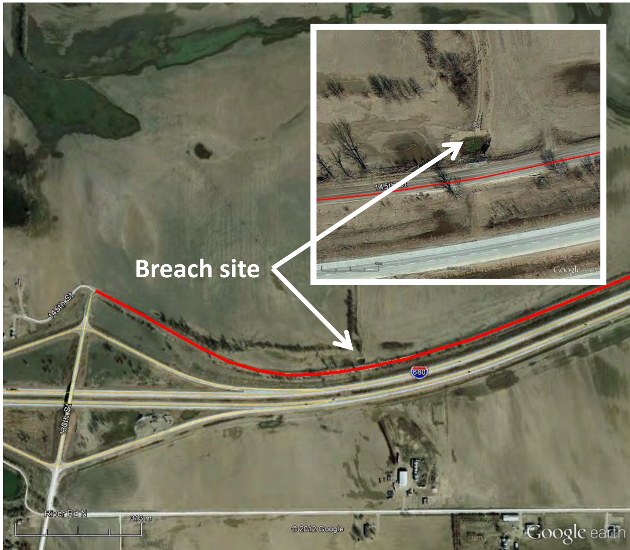
Figure 97. Aerial imagery of the breach site located next to TS5 145th St. (Google image from 3/7/12) – Pottawattamie County
