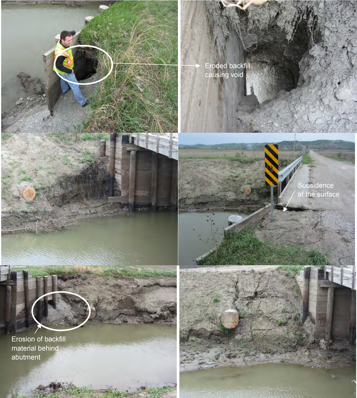
Figure 134. Bridge conditions on TS1 on 4/4/12 – Fremont County
