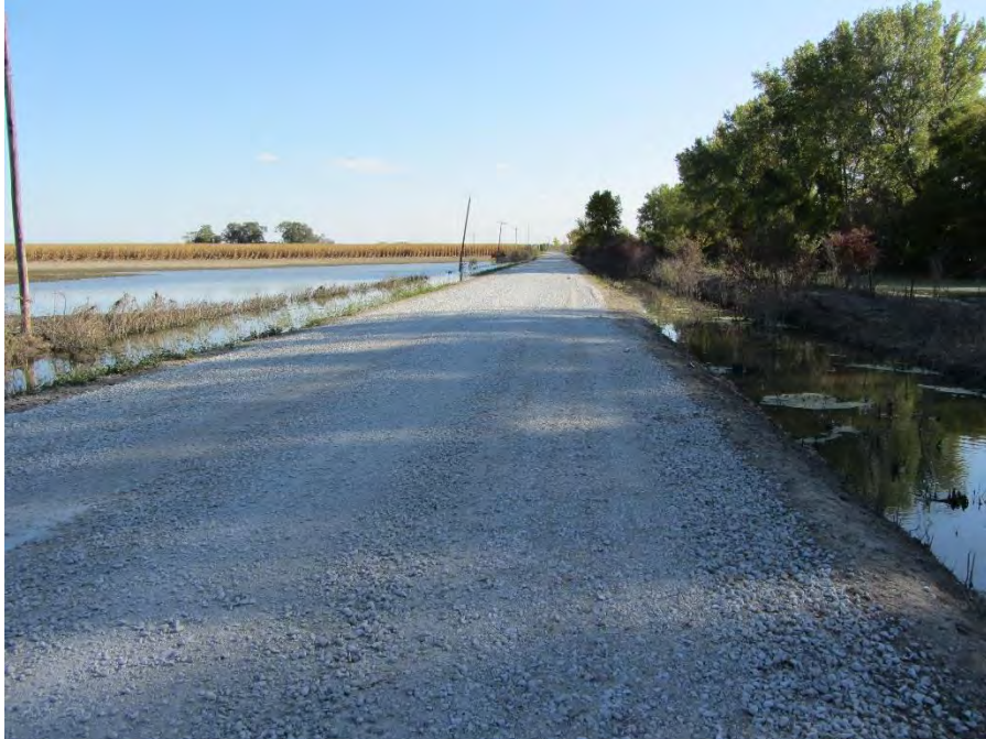
Figure 72. New gravel placed at the middle of the segment following flooding on TS3 (Photo taken on 9/21/2011) – Pottawattamie County
