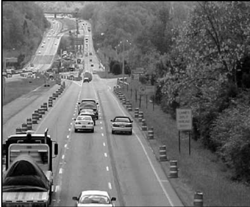
Figure 4.5. Work zone contra-flow concept utilized by ODOT (55)
