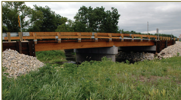
Demonstration bridge located in Delaware County, Iowa.
