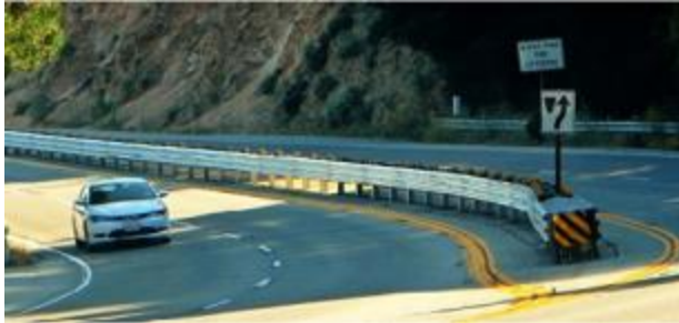
(c) Median W-beam barrier
