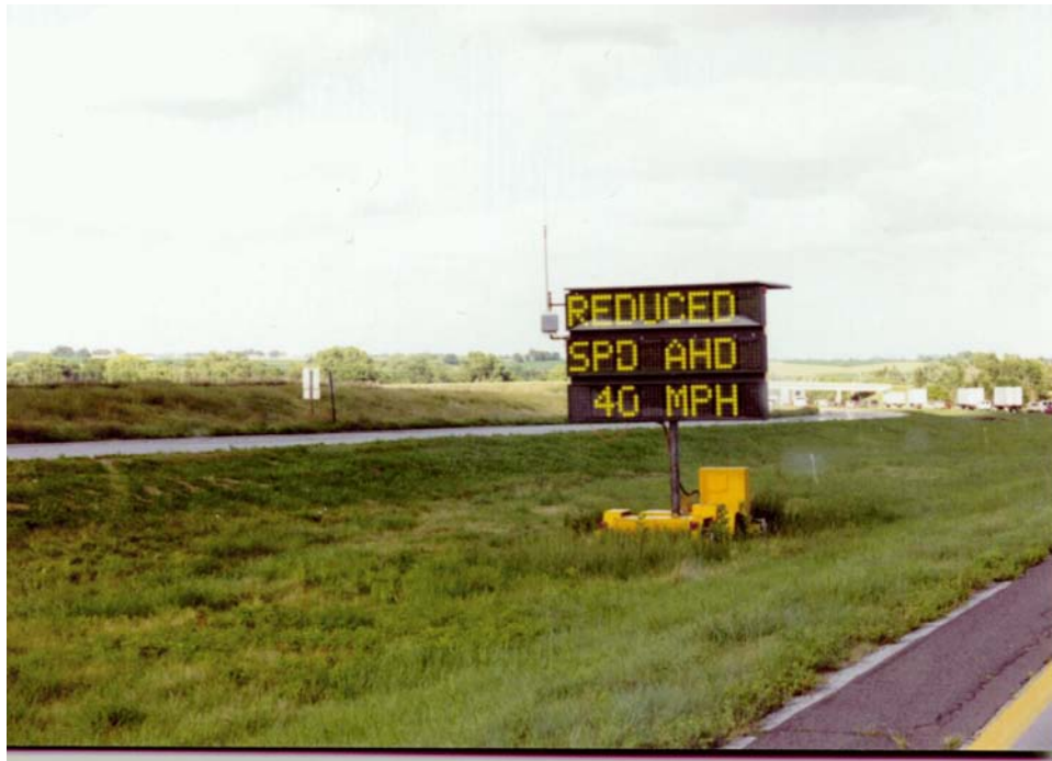
FIGURE 5-11 ADAPTIR VMS placement.
