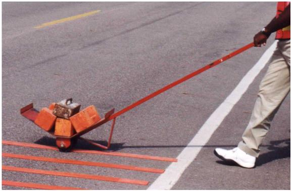
Figure 5. Tampering Card Used During Installation
