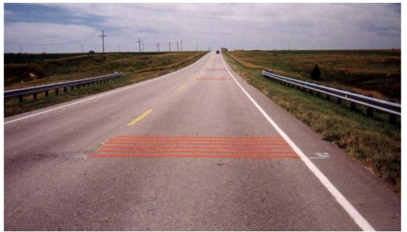
Figure 3. Removable Rumble Strip Evaluation Installation
