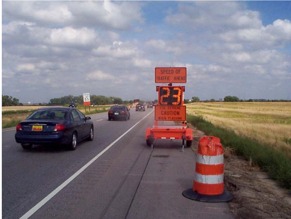
FIGURE 6 D-25 Speed Trailer in Operation close to the Work Zone
