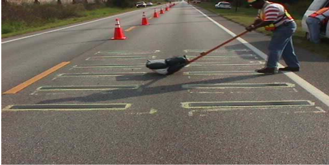
FIGURE 2 Installation of rumble strips with 200-lb roller
