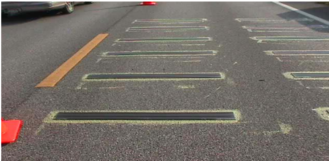
FIGURE 3 Driving lane after installation of the rumble strips
