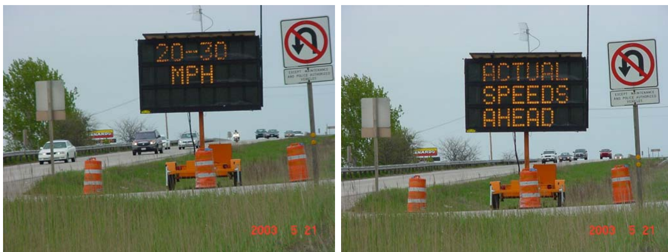
FIGURE 1 Two Alternate Messages Displayed by the Variable Message Sign, Located on the Median of US 41
