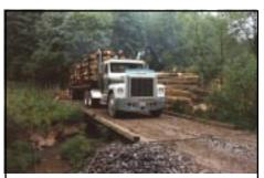
Utilization of a portable timber bridge
