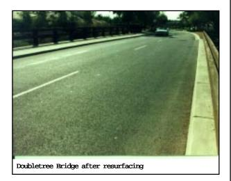
Summary: In conclusion, the asphalt rubber overlay system's increased flexibility has proven to be a moderate to exceptional solution to mitigate severe cracking in conventional asphalt concrete pavement overlays which reflect severe wood deck shrinkage movement, typical in the dry and torrid southwest Sonoran Desert.
