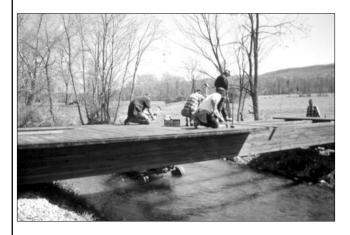
When all the panels had been secured, end walls were attached to each end of the bridge. From start to finish, a relatively inexperienced six man crew was able to complete the job in about 24 hours.
