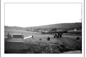
Three beams were required to meet the weight requirements of an H-10 design vehicle, which is a 10 ton, 2 axle truck. The design axle loads are 4,000 lbs. and 16,000 lbs. spaced 14 feet apart. This accommodates most small farm equipment and light truck traffic.
