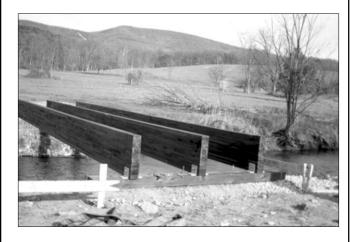
Next, the first glued-laminated deck panel was dropped into place with the loader. Successive panels were rolled into place using round steel bars. This method worked very well considering the weight of the panels, each measuring 3-1/8 inch x 4 feet x 12 feet.
