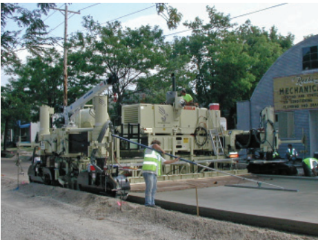
Urban concrete overlay construction with limited paving clearance (Photo courtesy of Kevin Klein, Gomaco)
