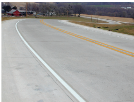
Completed concrete overlay of rural roadway with paved shoulders (Photo courtesy of Gordon Smith, P.E., Iowa Concrete Paving Association)
