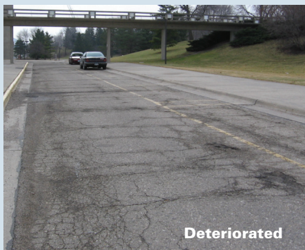
Figure 9. Examples of existing pavement conditions (Photo courtesy of Snyder and Associates)
