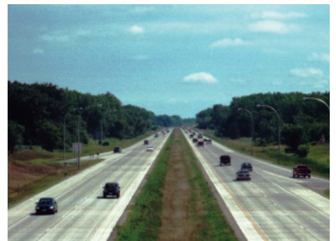
Completed concrete overlay on interstate highway (Photo courtesy of Matt Zeller, P.E., Concrete Paving Association of Minnesota)
