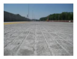
When specifying both longitudinal and transverse tining, texturing should be applied as soon as possible after finishing, but before the concrete has attained its initial set. This is accomplished by applying both a drag pretexture and subsequently by tining.
