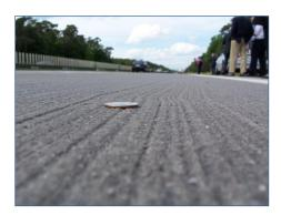
In order to assure uniformity, the turf must be mounted on a work bridge or a moveable support system that allows for adjustment of the area of turf in contact with the pavement. A single piece of turf spanning the full width of the pavement must be used. To achieve the desired texture, a minimum length of 5 ft. of turf must be in contact with the concrete at all times.
