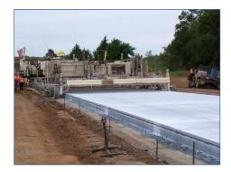
For both drag (CPSCP GS-2) and tined textures (GS-3 and GS-4), the protection of the concrete surface is of paramount importance. Unless proper methods of curing are adopted, the texture can deteriorate prematurely under the influence of traffic and climate.
