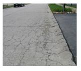
network of multiple, closely spaced cracks, often accentuated with staining or deposits. However, visual inspection alone cannot confirm the presence or absence of material-related issues. Laboratory testing of pavement core samples is required to definitively confirm the mechanisms that may be contributing to distress.
