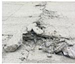
can be dramatically released as the pavement thrusts upwards and/or shatters. Contributing factors are incompressible in the joint, high coefficient of thermal expansion (CTE) of coarse aggregate as the concrete temperature increases, and long transverse joint spacing.
