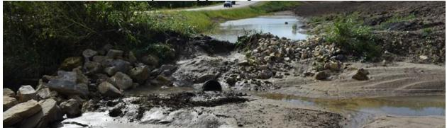
(d) Washout of berm, riser pipe discharge elevation higher than inflow, sedimentation prior to dewatering
