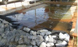
(c) Riprap ditch check w/ 8 oz FF choker Figure 4.28. Riprap ditch c
