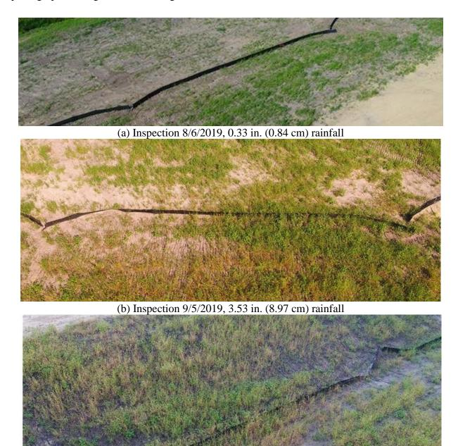
(c) Inspection 9/24/2019, 6.78 in. (17.22 cm) rainfall Figure 5.7. Standard silt fence perimeter control aerial inspection photos
