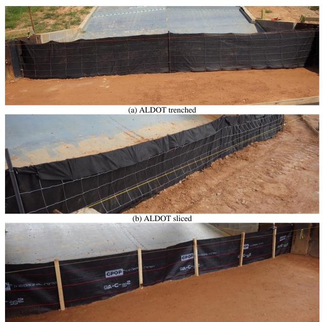
(c) AL-SWCC Figure 5.2. Alabama silt fence configurations
