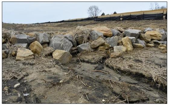
Figure 4.30. Rock check dam undercutting
