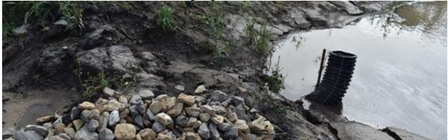
(b) Erosion of overflow berm
