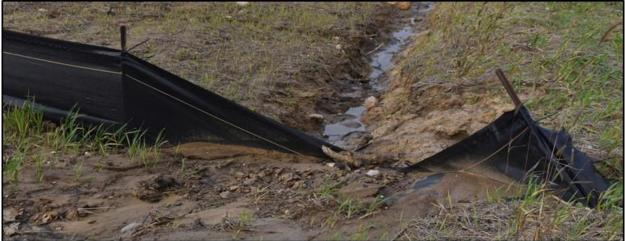
(c) Flow bypass of silt fence ditch check Figure 4.14. Silt fence ditch check failures
