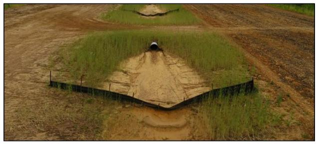
Figure 4.13. Silt fence ditch check overtopping due to T-post deflection
