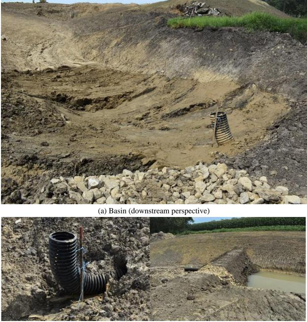
(b) Riser pipe structure (c) Spillway Figure 6.2. Typical sediment basin installed in Tama US 30
