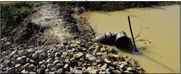
(b) Sample float system at discharge Figure 6.8. Single sediment basin sampling locations and dewatering system
