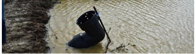
(c) Buoyant riser pipe dislodged from basin bottom
