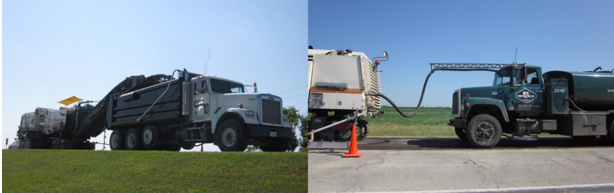
Figure 7. Pavement scarification operation
