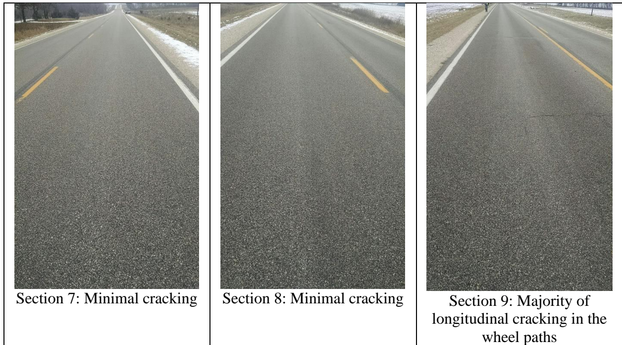
Figure 24. Post- construction conditions of treatment sections
