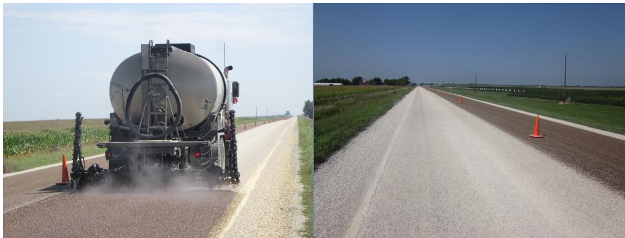
Figure 15. Dust control for seal coat
