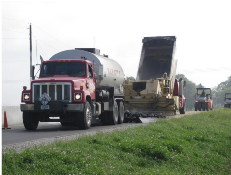
Figure 14. Construction of seal coat
