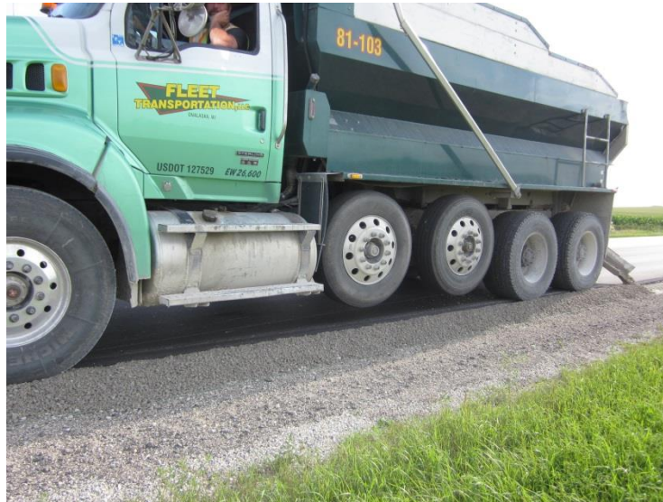
Figure 16. Shoulder aggregate placement vehicle
