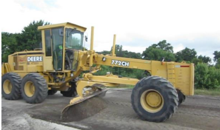
Figure 12. Motor grader used for finishing FDR
