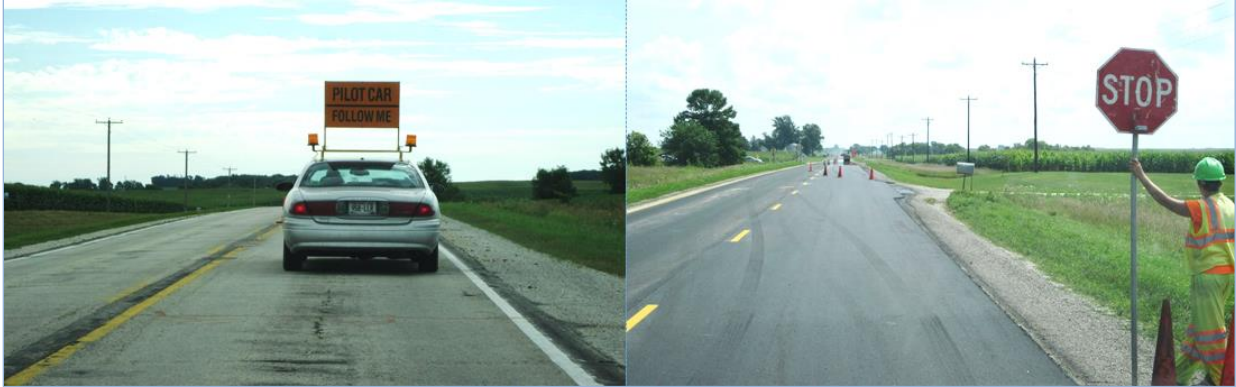
Figure 17. Single-lane pilot car traffic control
