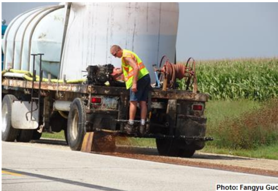
Figure 33. Paved road protection from soapstock splashing
