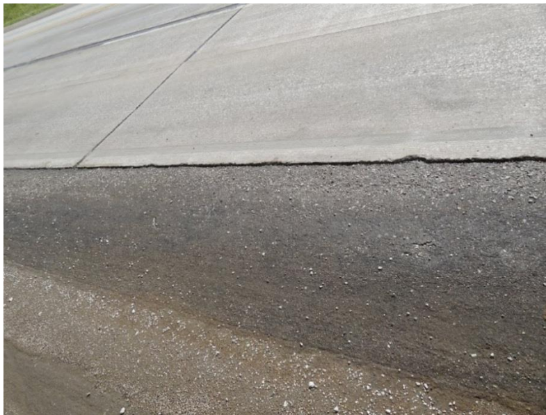
Figure 20. Southbound shoulder of US 169 south of Algona, Iowa
