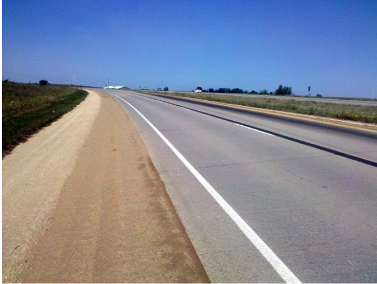
Figure 13. Soapstock and sand applied on the shoulder of US 63 near Denver, Iowa
