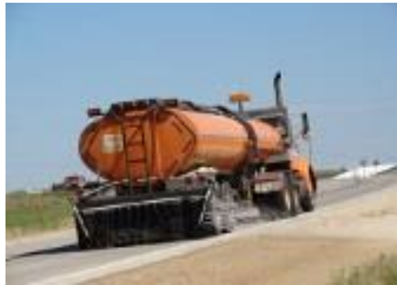
Figure 36. Water truck moistening the shoulder
