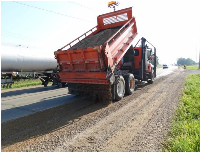
Figure 10. Sand applied on the shoulder of US 18 near Garner, Iowa
