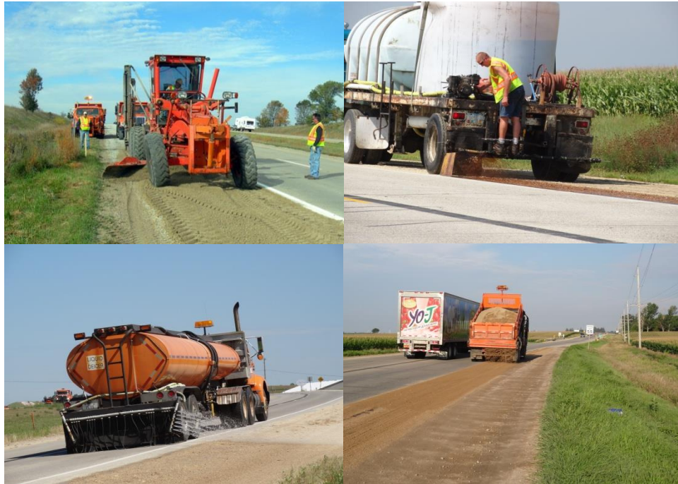
Figure 5. Road grader (top left), soapstock truck (top right), water truck (bottom left), and sand truck (bottom right)
