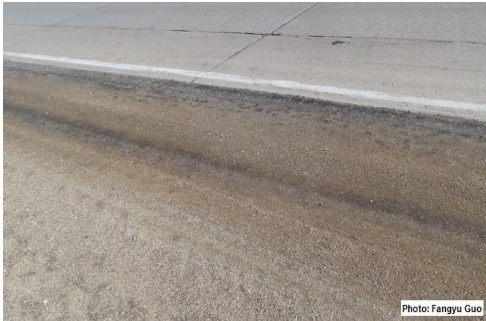
Figure 38. Shoulder after soybean soapstock application
