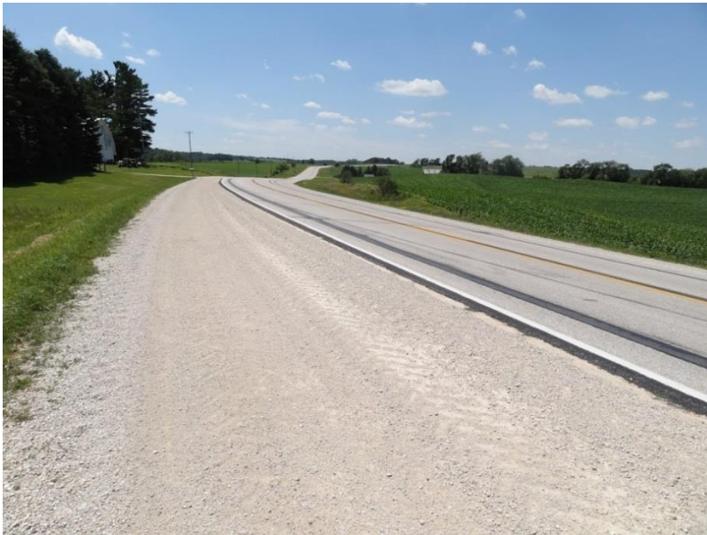
Figure 29. Shoulder of US 18 on eastbound west of Clermont, Iowa
