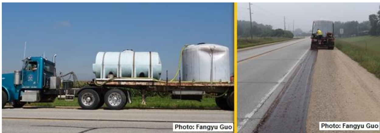
Figure 37. Application of soybean soapstock over the granular shoulder
