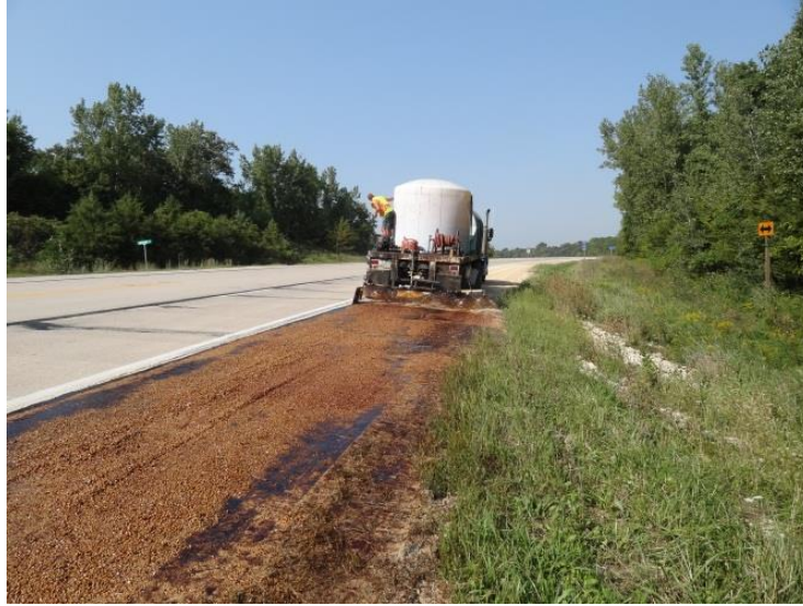
Figure 15. 12 ft wide soapstock applied on the shoulder of IA 13 east of Elkader, Iowa
