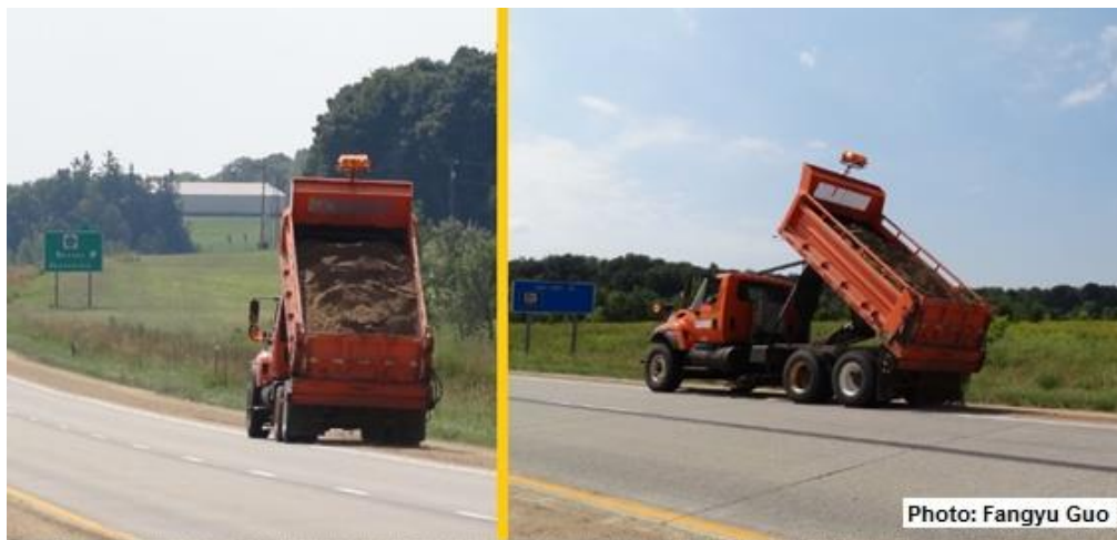
Figure 39. Truck spreading sand over the treated granular shoulder
