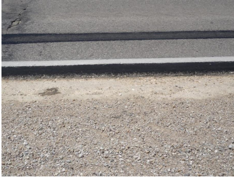
Figure 28. Shoulder of US 18 eastbound east of West Union, Iowa
