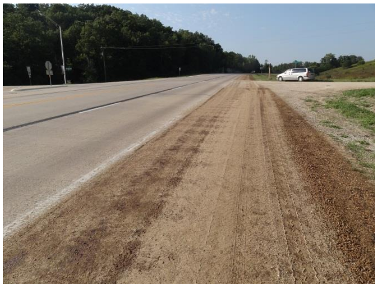
Figure 16. Sand applied on the shoulder of IA 13 east of Elkader, Iowa
