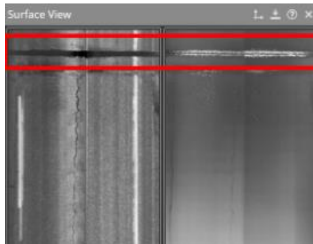
Figure 20. Road surface at bridge entrance expansion joint
