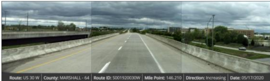
Figure 21. Bridge 6485.3L030 entrance view
