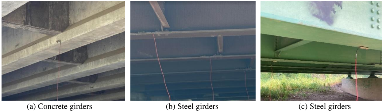
Figure 7. Strain gauge mounting techniques
