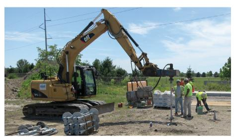
Helical pile installation equipment
