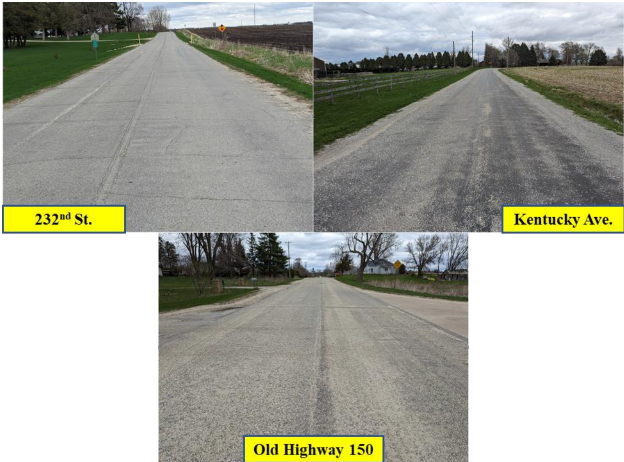
Figure B2. Otta seal site appearance in Buchanan County (photos taken on April 21, 2023)
