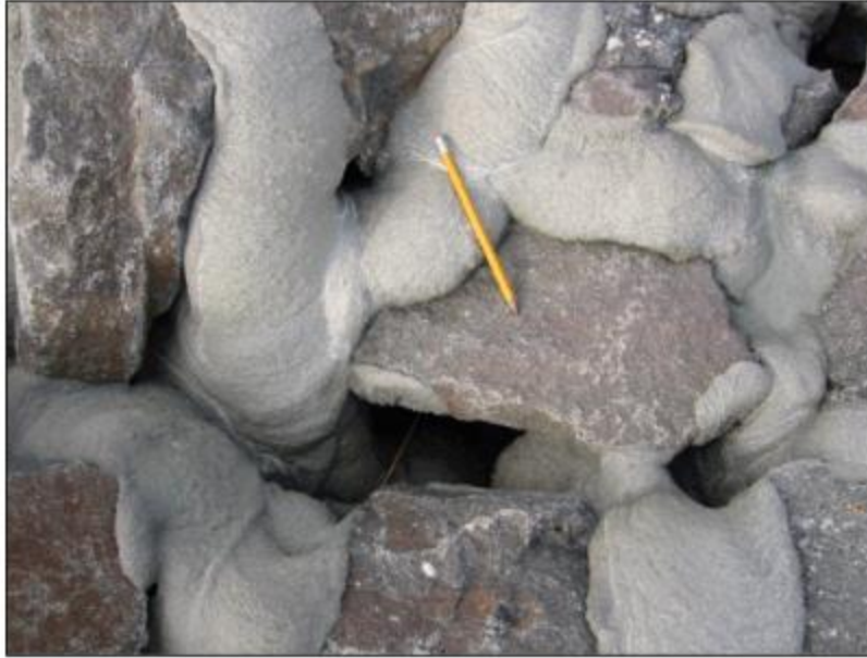
Figure 7. Partially grouted riprap
