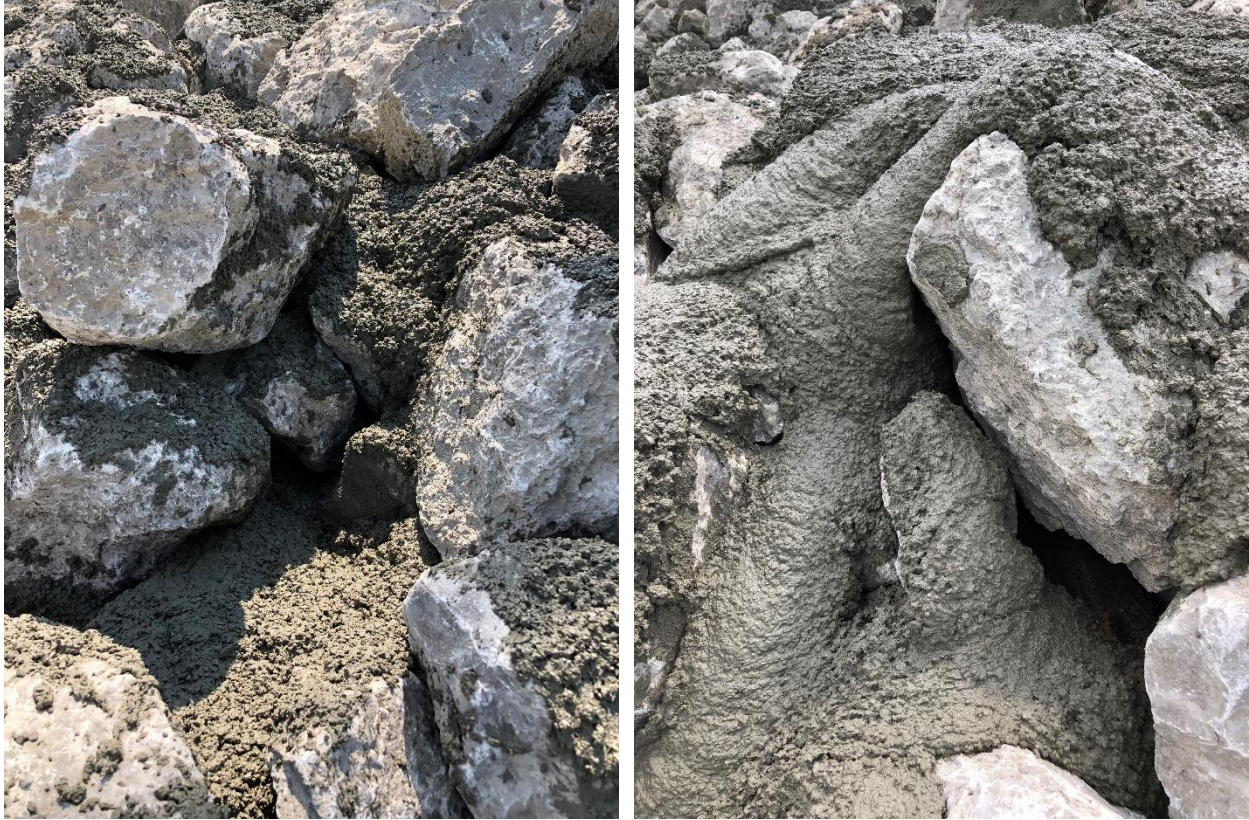
Figure 42. Initial grout consistency (left) and desired grout consistency (right) in Wayne County
