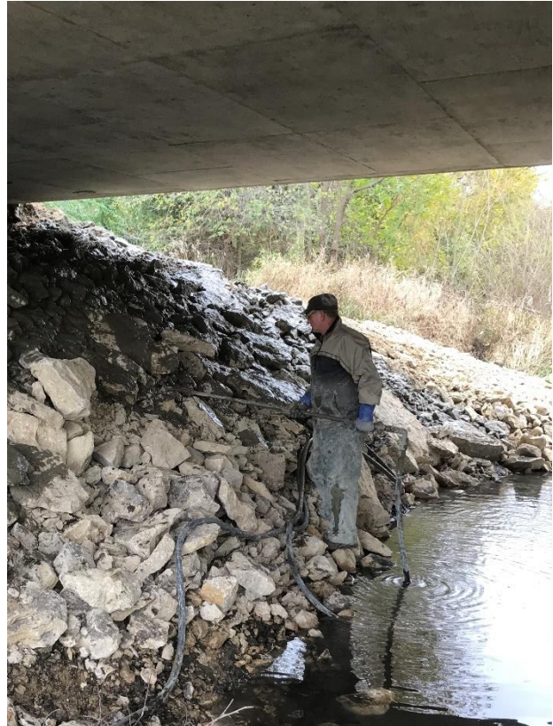
Figure 35. Grout placement of FHWA mix (left) and Buchanan County grout (right)
