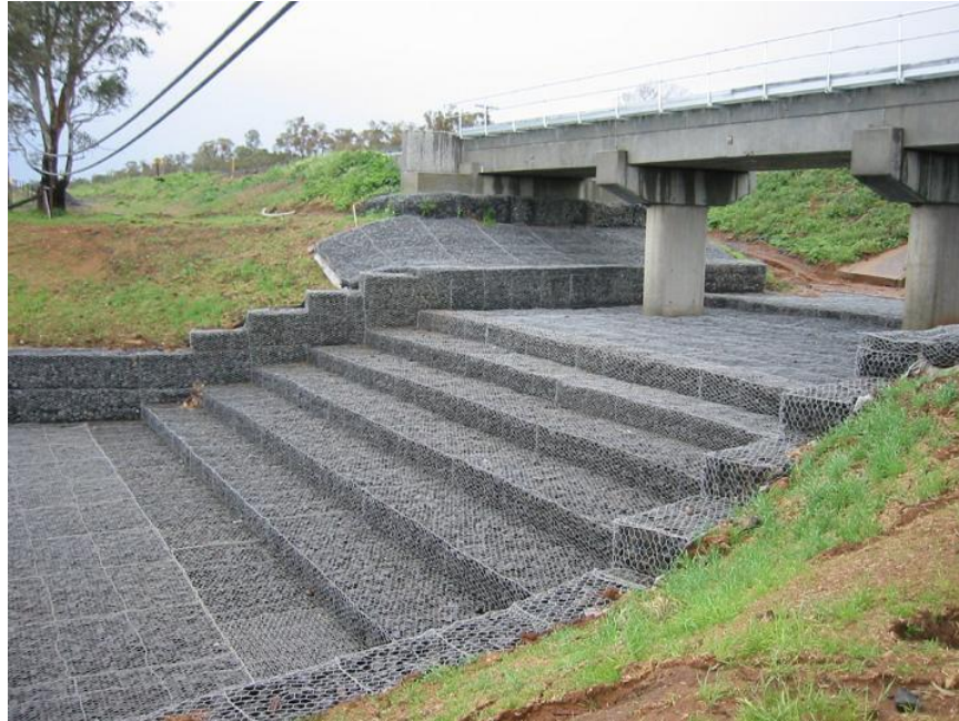
Figure 11. Gabion mattress after installation
