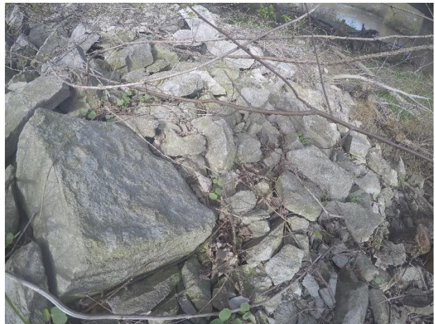
Figure 31. Undersized loose riprap in Madison County, Iowa
