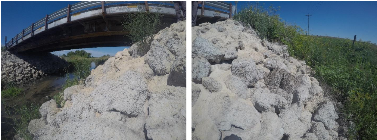
Figure 28. Grouted riprap in Buchanan County, Iowa
