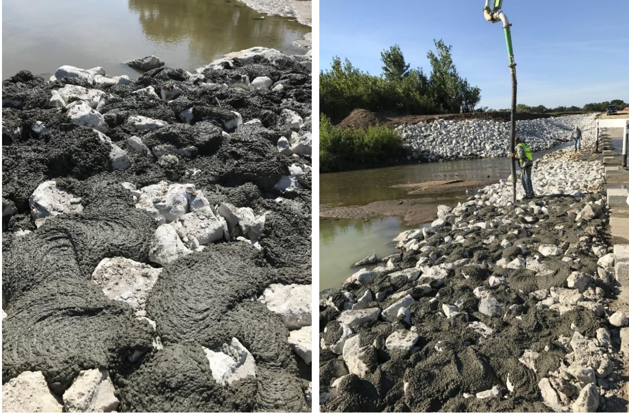
Figure 38. Madison County pilot installation grouting
